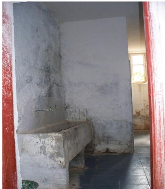
Figure 13: The sink of the first floor restroom.
