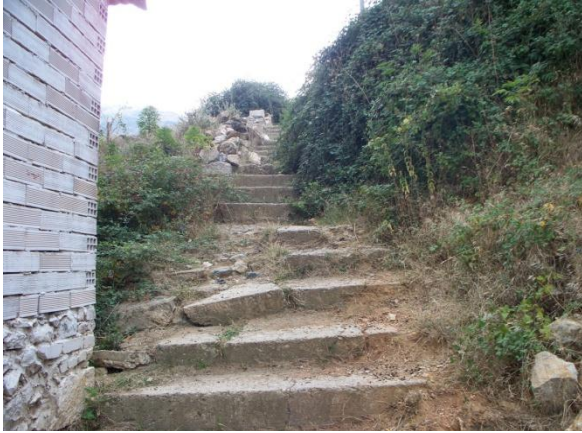
Figure 8: The main stairs of the school.
