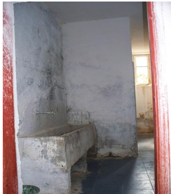
Figure 13: The sink of the first floor restroom.
