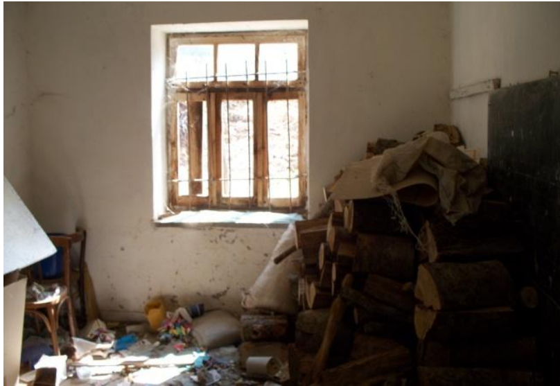
Figure 8: The firewood used for heating at Kuç i Zi School.
