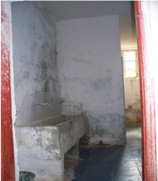
Figure 13: The sink of the first floor restroom.
